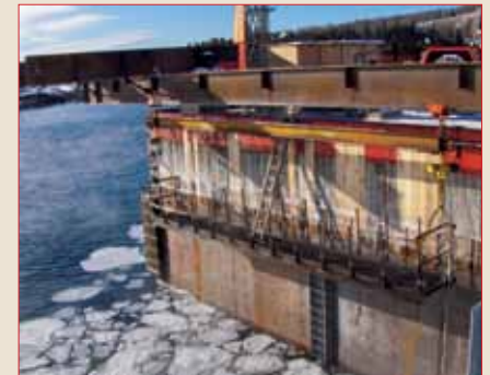
Wharf renovation project at the Escoumins boarding station.
